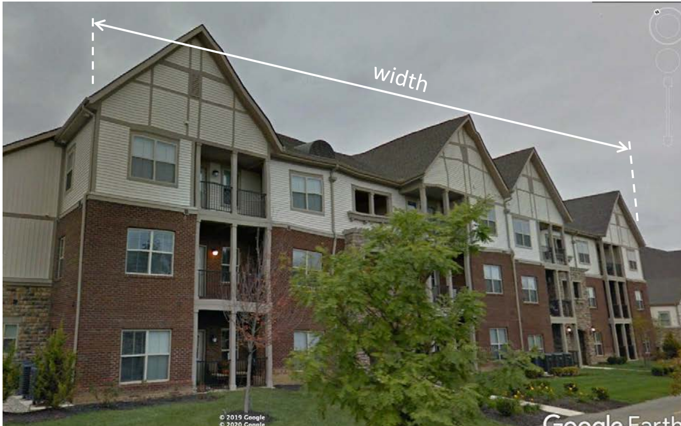
Conventional Apartment Project
